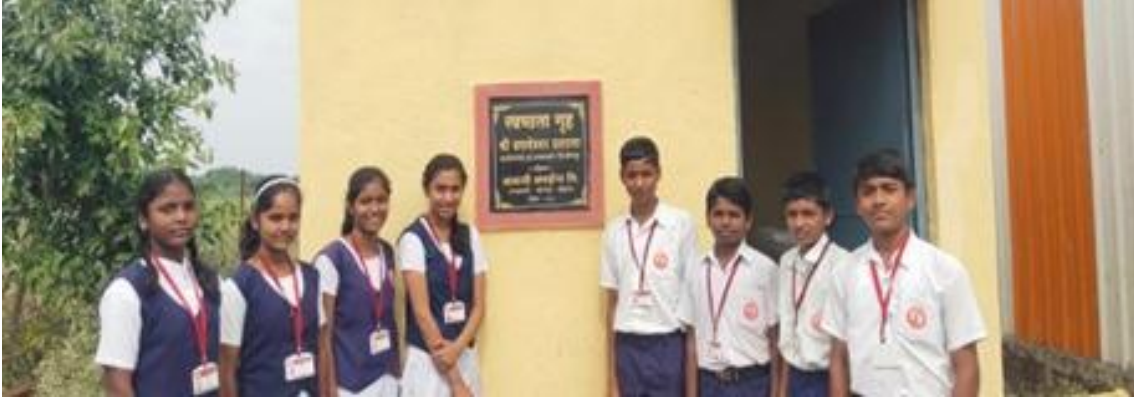
Constructed Toilet Block at Shree Basaveshwar Prashala, Kazikanbas dt 31.01.2024
